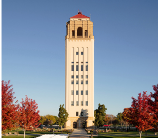
Unity Tower - Awaken Whole Life Center Exterior Restoration/Rehabilitation Unity Village, Missouri
